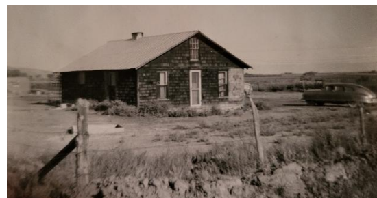
Figure 10 The original house at Loma – it had a 'tin' roof – I loved to hear the rain tap on it
