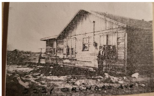
Fig 2 Original House at 2221 Orchard Ave, 1944
